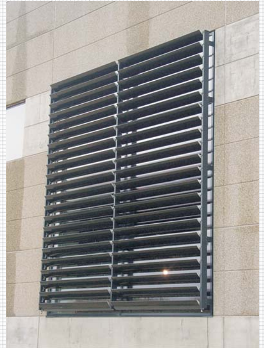
Building: Radin, Sveta Nedelja Aluminum brisoleys
