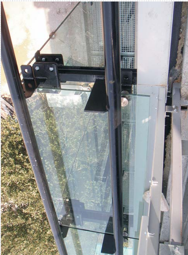
Building: VIP, Spider facade - glass corner
