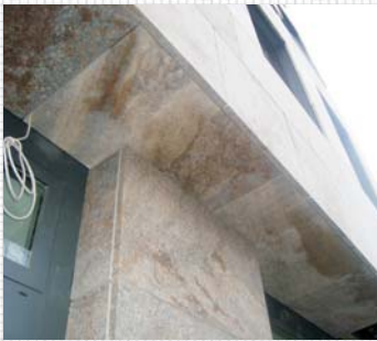
Building: Maksimir, Zagreb, Stone cladded ventilated facade
