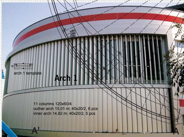
Building: VIP kindergarden, Žitnjak, Zagreb Aluminum briseleys
