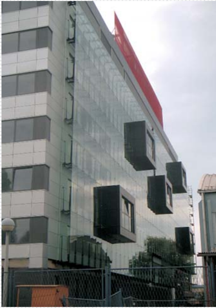
Building: VIP, Žitnjak, Zagreb Spider facade
