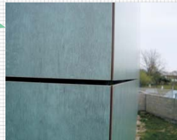
Detail of two ventilated facades junction
