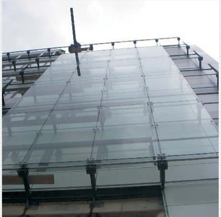
Building: VIP, Žitnjak, Zagreb Spider facade
