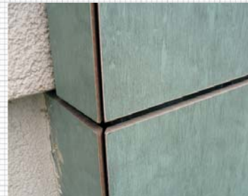
Detail of ventilated and ETICS facades junction
