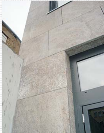
Building: Maksimir, Zagreb, Stone cladded ventilated facade
