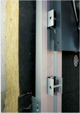
Detail: hanging the ACP cassette onto aluminum subframe
