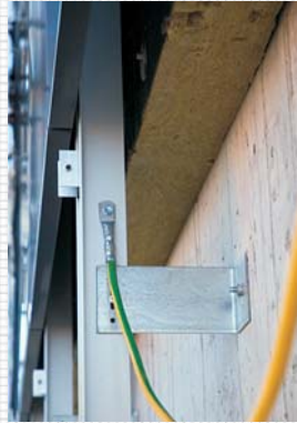
Detail: earthing of the aluminum subframe
