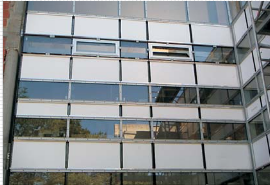
Building under construction
